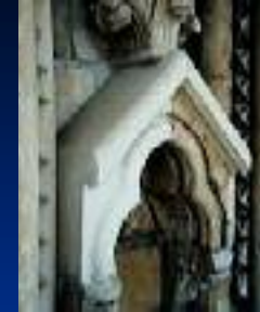
Correct alignment between new and old masonry
